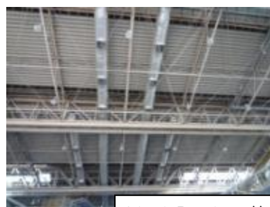
No.1 Dock 天井
